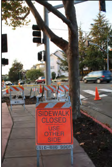
New signal installation, Rose and Grand
