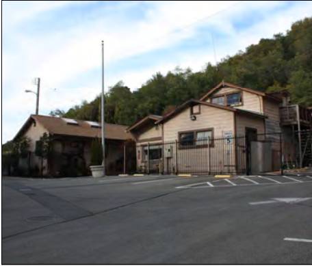
Piedmont Corporation Yard, Moraga Avenue
